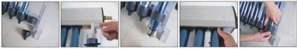
**Step1:** First install the nylon cap on the bottom track, and then screw off the jacket from the nylon cap.
